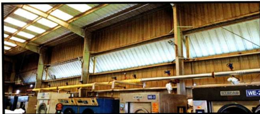
Pic. 53 Steam Condensate Collection Pipeline
