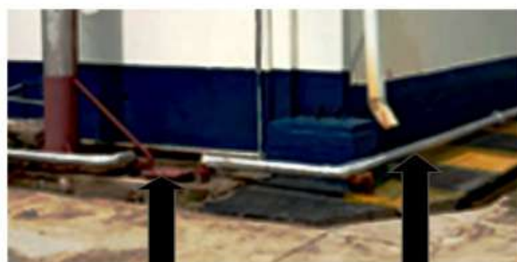
Pic. 53 Steam Condensate Collection Pipeline
