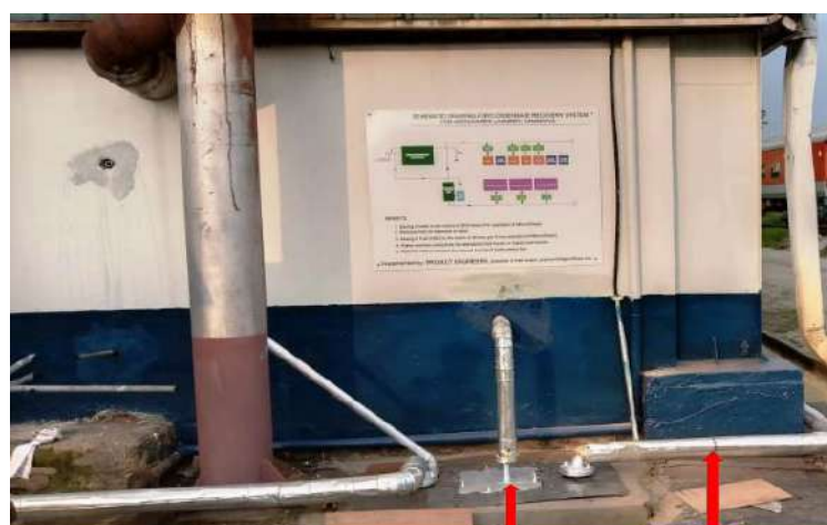
Pic. 53 Steam Condensate Collection Pipeline
