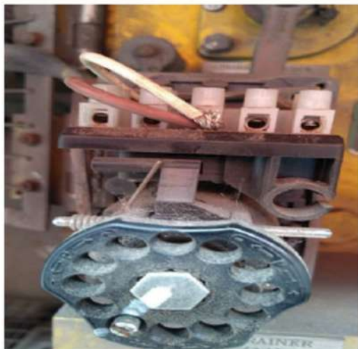
Figure-14 (defective pressure switch)
